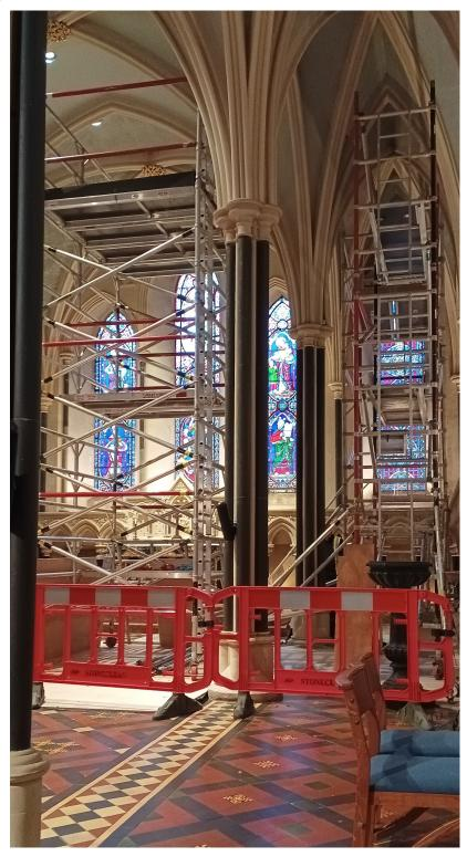
Ongoing works in the lady chapel to restore the roof which involves cleaning and repainting. Conservation & Restoration are charged with this work.
